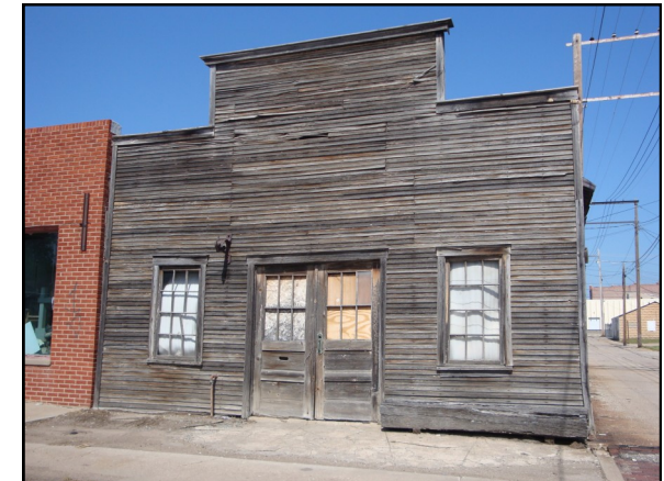
BEFORE Façade Grant
